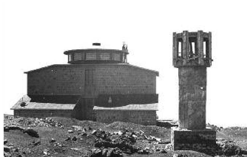
February 24, 1947. The Etnean Observatory after the end of the restoration work begun in 1939 which led to the dismantling of the old dome and the construction of the meteoric tower.
